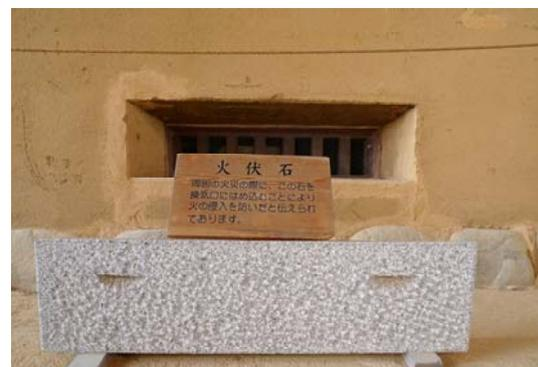
**Figure 2(B).** Fire suppression stone used in the Edo period barns
