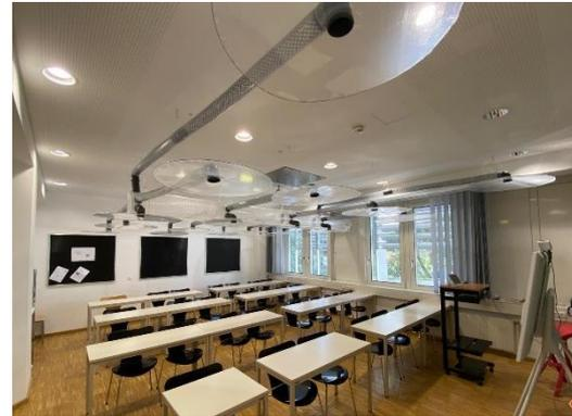
Figure 1: Max Planck Institute (MPIC)- Mechanical Extract Ventilation (MEV) system installed in a TU Graz seminar room
