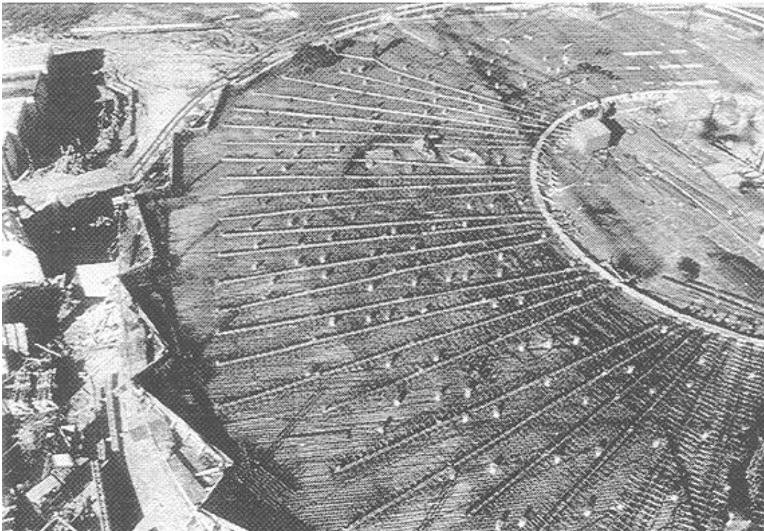
Inserted ceiling shuttered with armouring and intake supply ducts (ventilation, electronic data processing)
