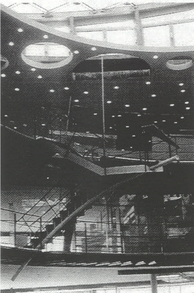
Inserted ceiling shuttered with armouring and intake supply ducts (ventilation, electronic data processing)
