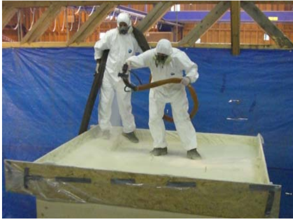
Figure 9: Spraying the foam insulation on the experimental set-up
