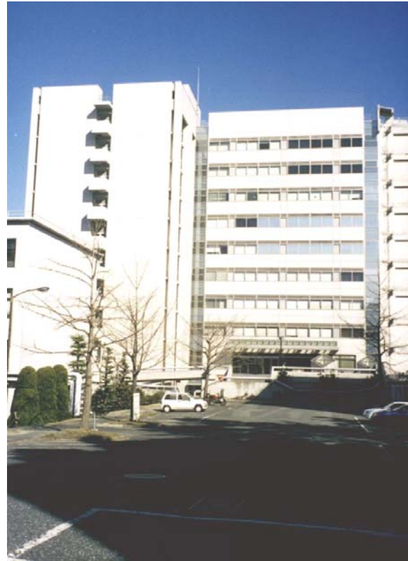
Figure 2 South face of case study building
