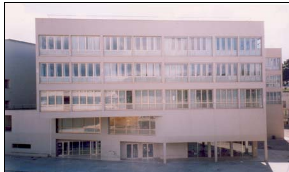
Figure 1. View from the South side of the building.
