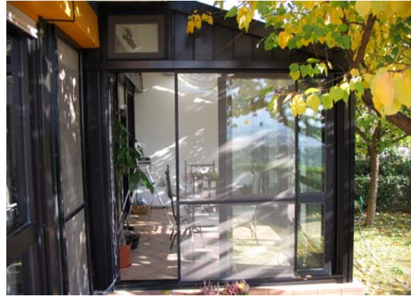
Fig. 3- external view of the greenhouse
