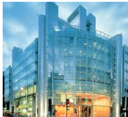
Figure 2 The Helicon building
