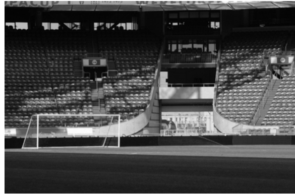
Figure 3 One of the four openings in the corners of the stadium with a surface area of 42.5 \text{ m}^2 .
