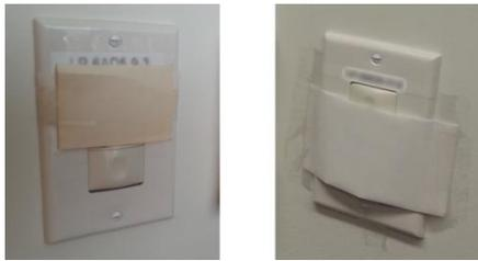
Figure 1. Evidence of taping occupancy sensor of light switch by occupants in an office building (taken from (Gilani and O'Brien, 2016)).
