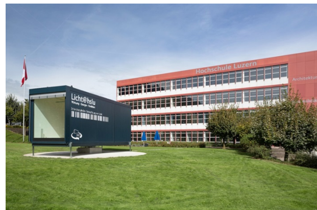
Figure 2: External view of the lighting/daylighting measurement container on the campus
