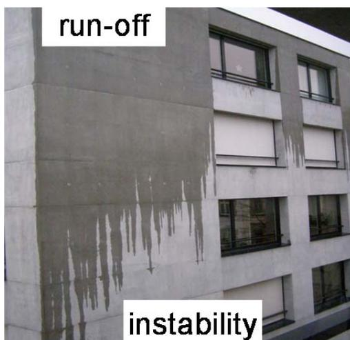
Figure 1: Rain deposition on building façade displaying also film forming and run-off on concrete façade during rain event.
