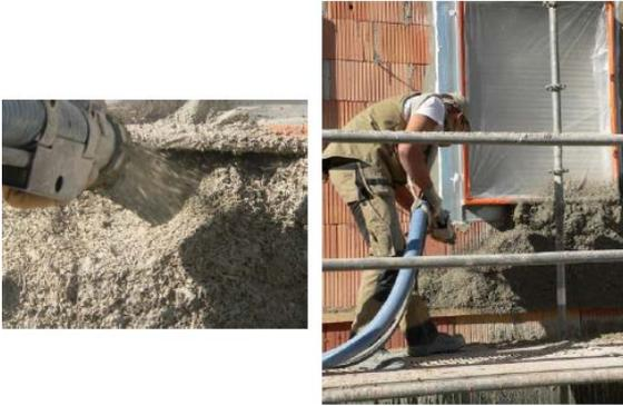
Fig. 1 – Hemp-lime concrete for building applications
