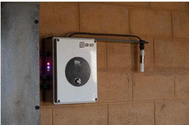
Figure 2 An IoT Box installed at a room level
