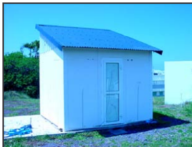
Figure 3: La cellule LGI
