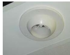
Figure 2a Nozzle diffuser
