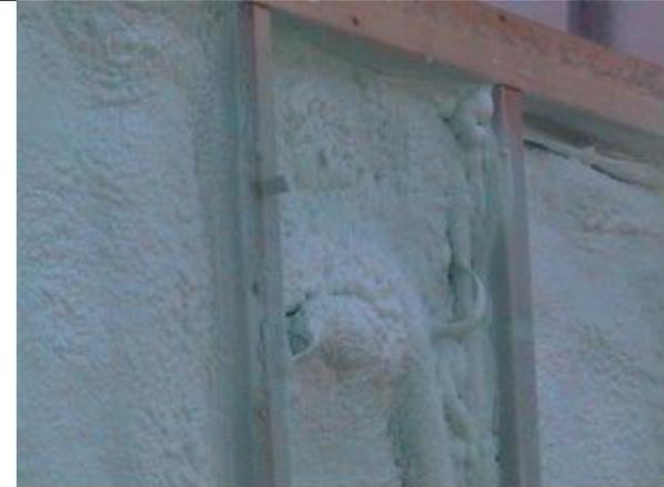
**Figure 8. Uneven SPF insulation thickness in WER 3A**
