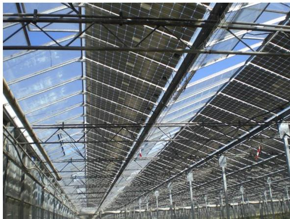
**Fig. 1:** STPV modules covering south-facing roof of a greenhouse in Montélimar, France (Tritec, 2015).
