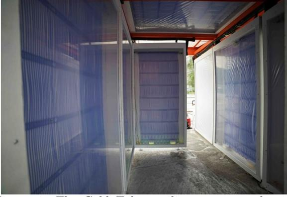
Figure 1: The Cold Tube pavilion constructed using 10 condensation free radiant cooling panels (Teitelbaum et al. (2019)).
