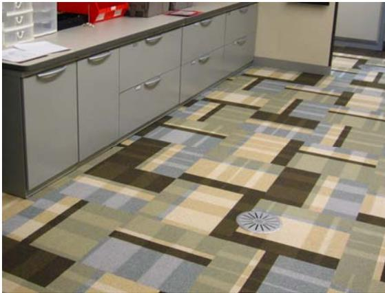
Figure 2: Under-floor air distribution in CDC
