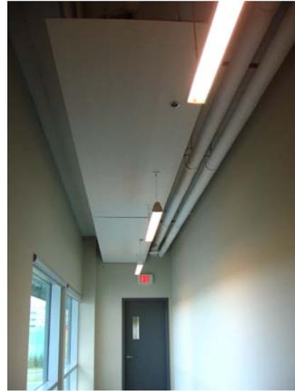
Figure 3: Radiant cooling panel in CDC (daylighting controls commissioning still in progress)
