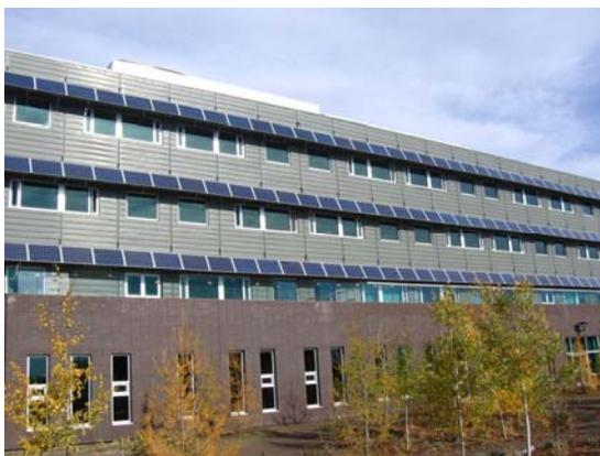
Figure 4: CDC BIPV system on south façade
