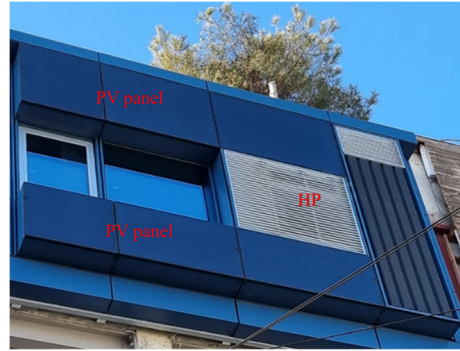
(b) Exterior view
