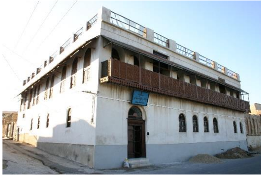
Figure 8- Tabib mansion in Bushehr, Source: Authors photography archive
