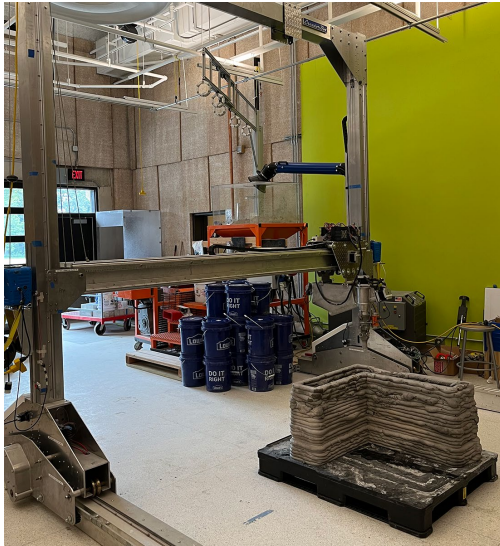
Figure 12 The full-size concrete wall printed with the Erectorbot 3D concrete printer
