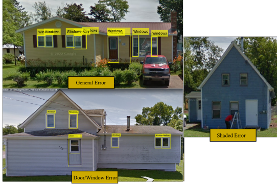
Figure 8: Common errors in facade identification
